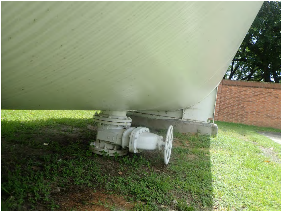
Photo 2: Bottom of tank with staining
