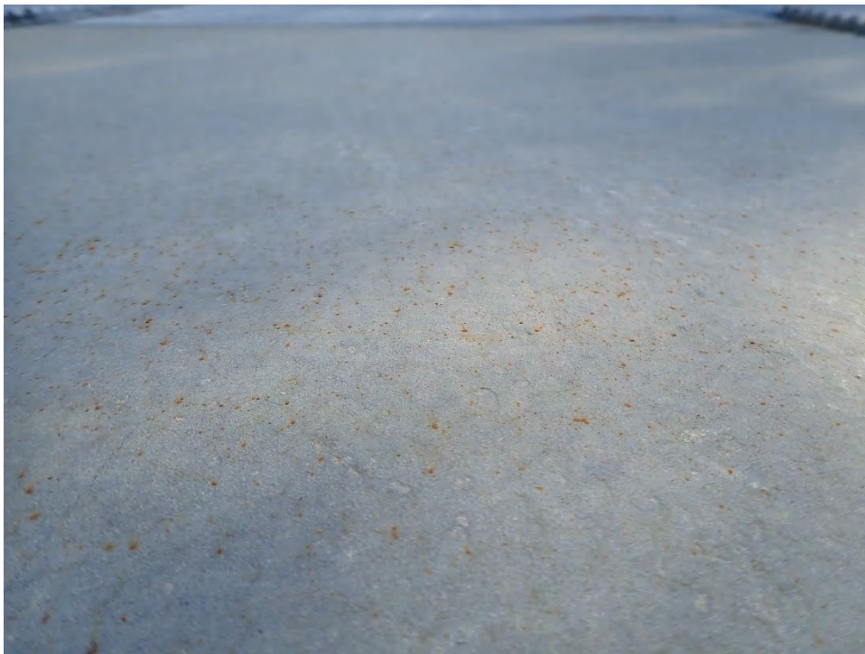
Photo 8: Roof with corrosion
