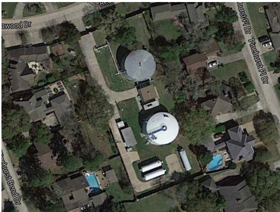
Water plant site overall
