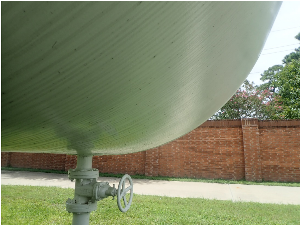
Photo 2: Tank with staining
