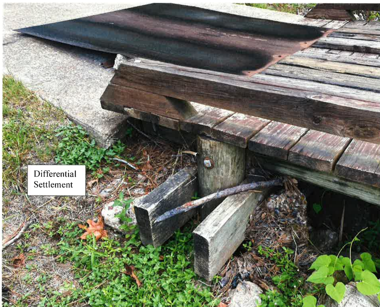
Figure 3 - Differential Settlements at the Bridge Approaches
