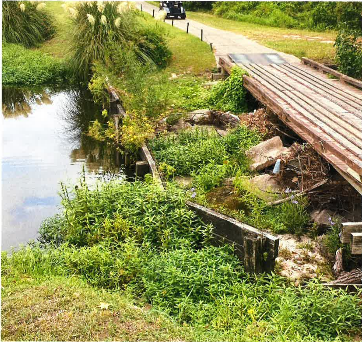
Figure 4 - Timber Weir Structure Overview
