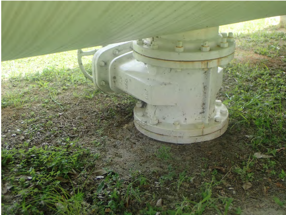
Photo 3: Inlet/Outlet line with corrosion
