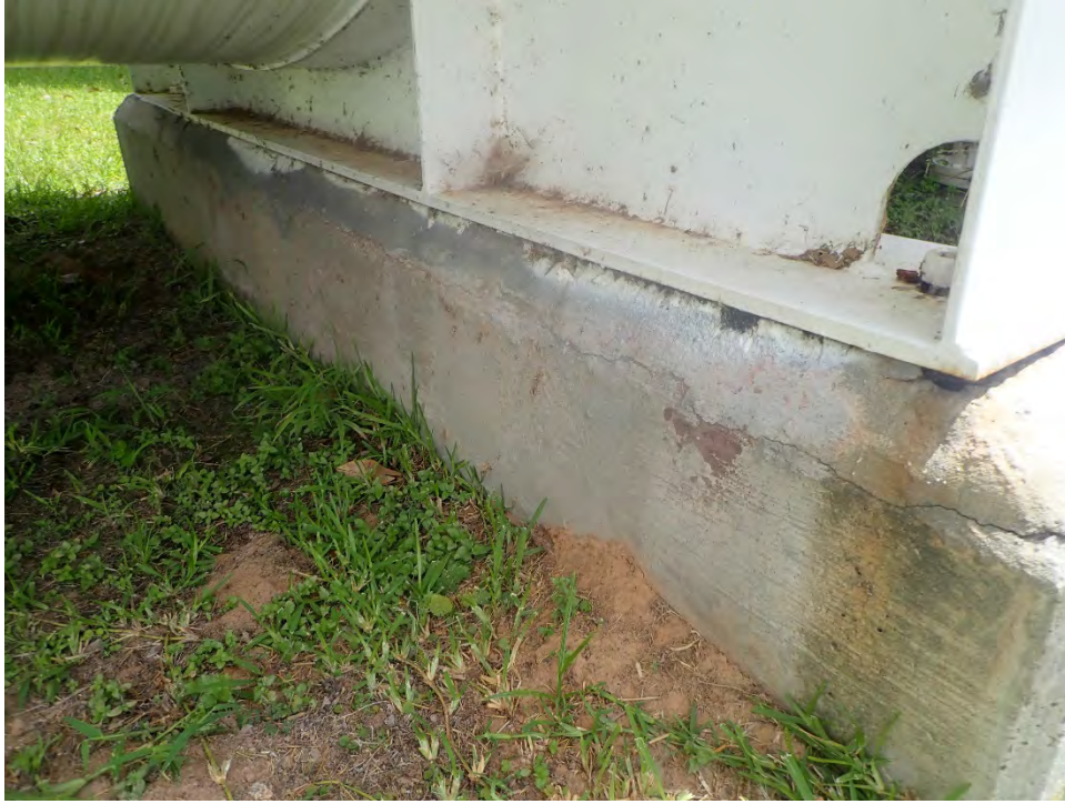
Photo 1: Concrete tank footing with cracking
