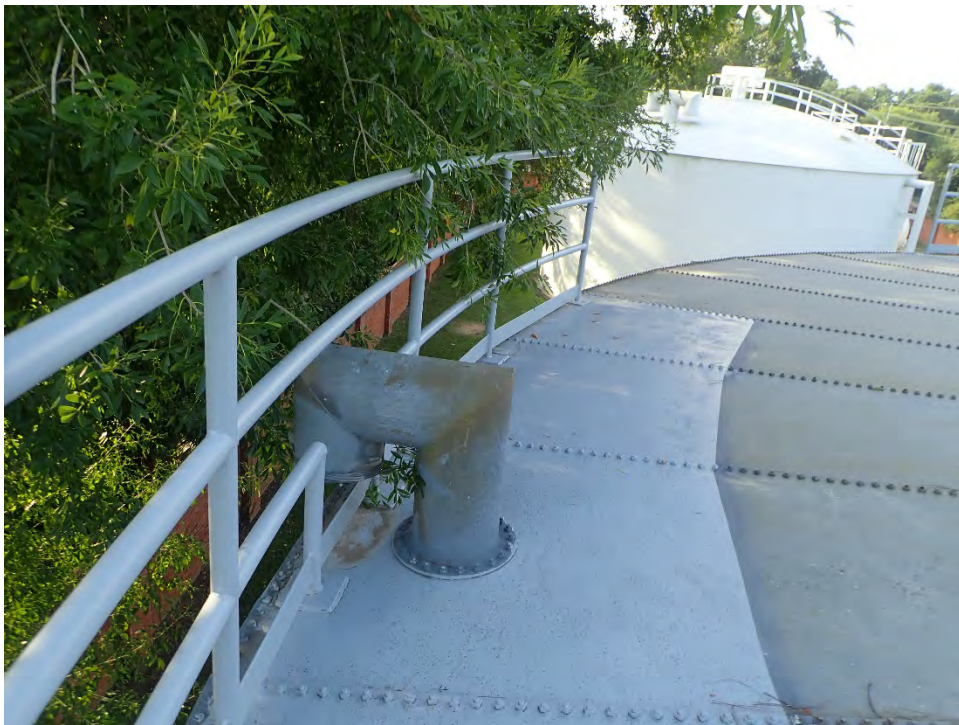
Photo 12: Roof hatch with corrosion
