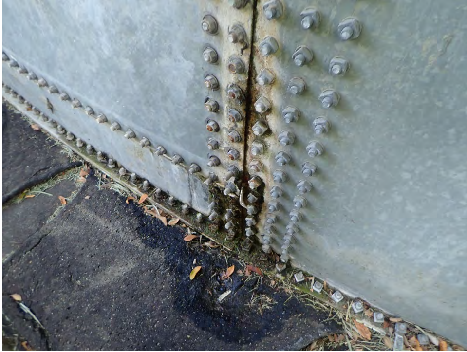
Photo 3: Side hatch with leak
