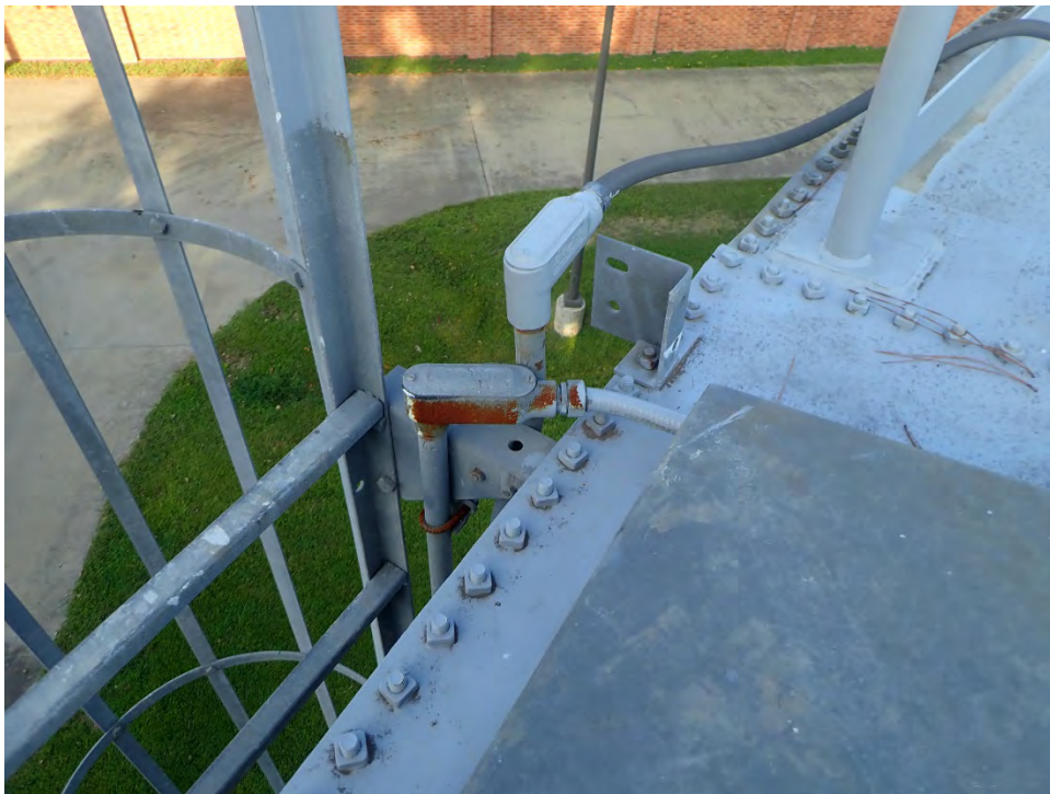
Photo 10: Electrical components with corrosion
