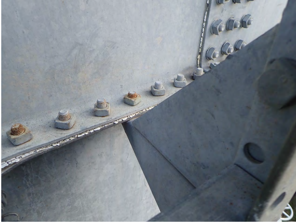
Photo 1: Tank sidewalls with corrosion
