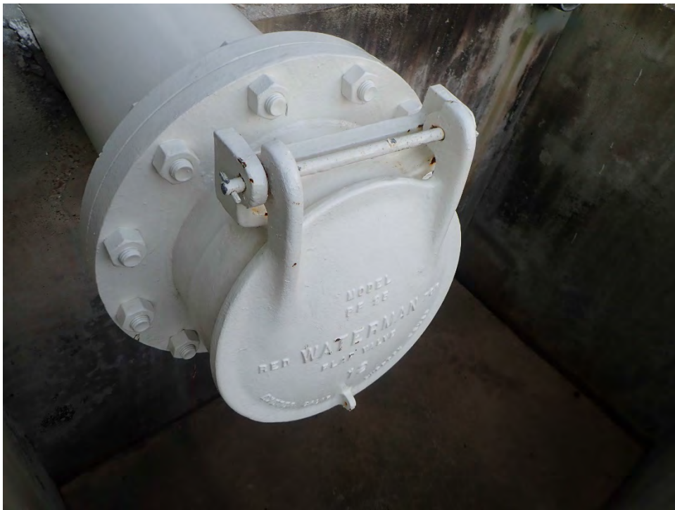
Photo 6: Drain line with corrosion
