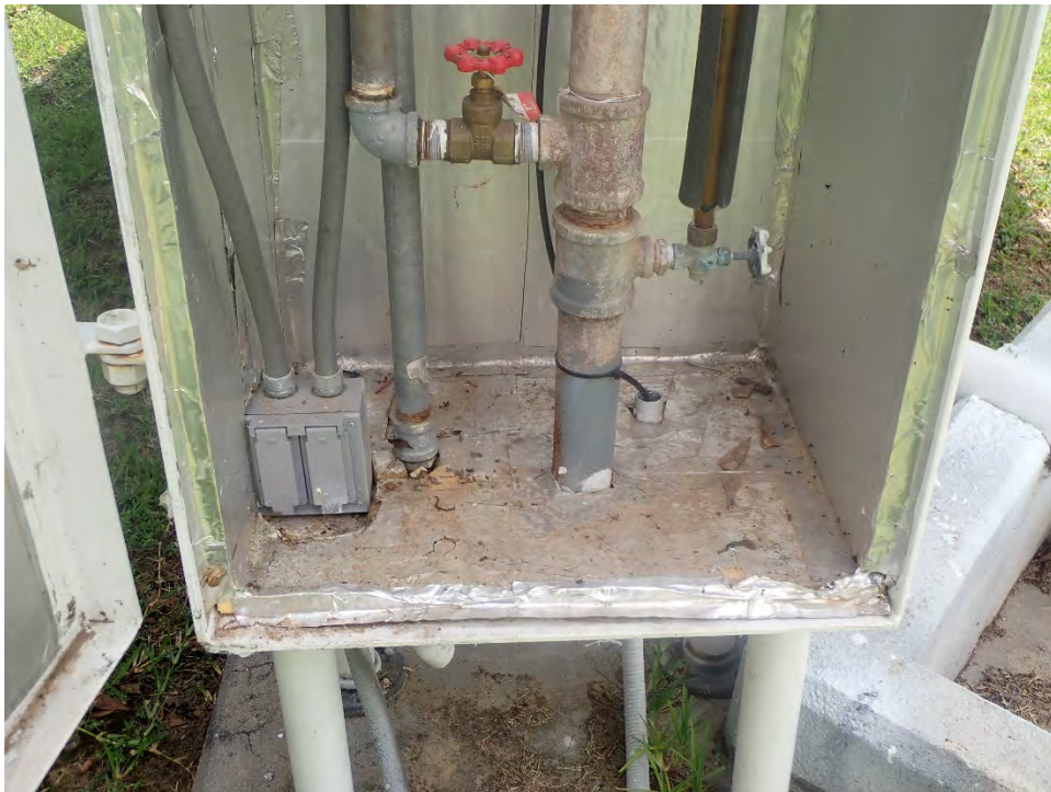
Photo 4: Equipment box piping with corrosion
