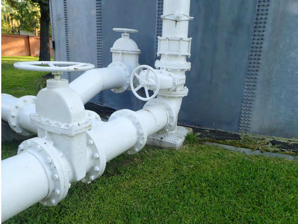
Photo 7: Fill line with corrosion
