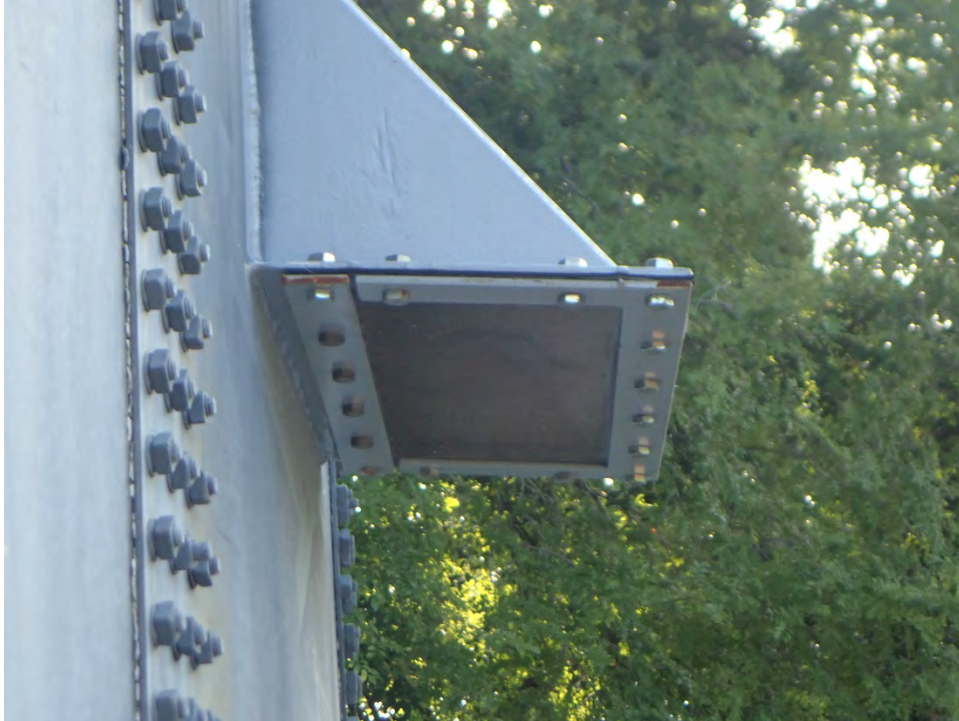
Photo 11: Shell vent with corrosion
