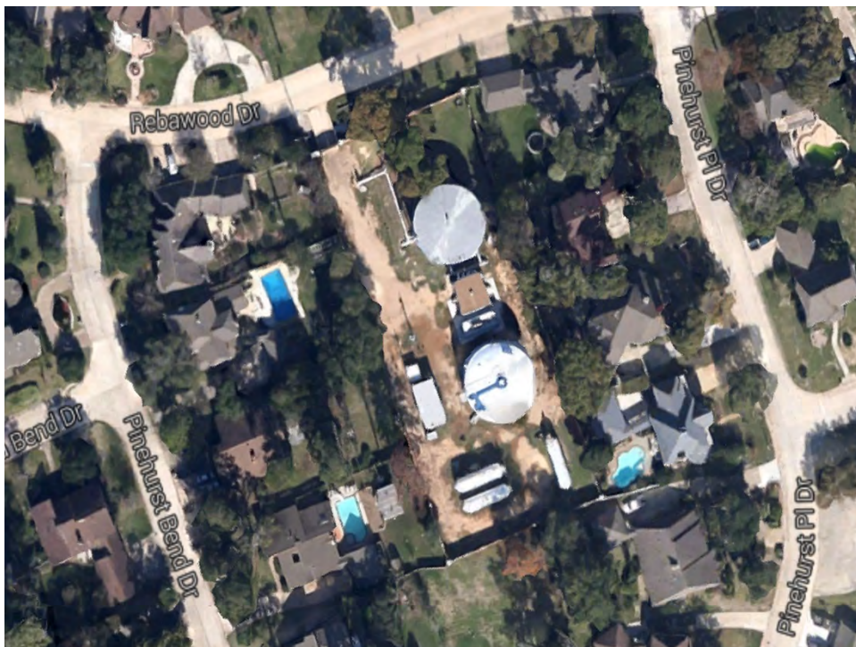
Water plant site overall
