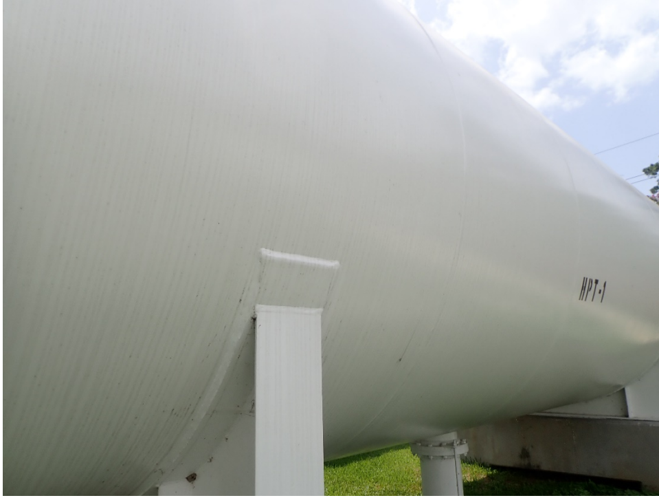
Photo 1: Tank with staining
