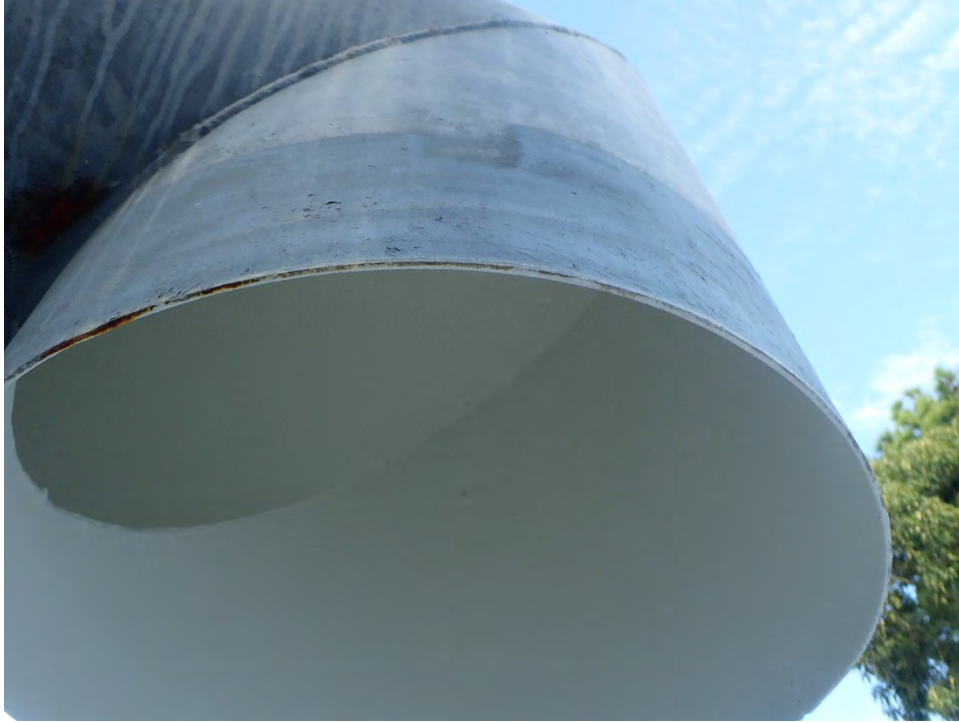
Photo 13: Roof vent with corrosion and missing screen
