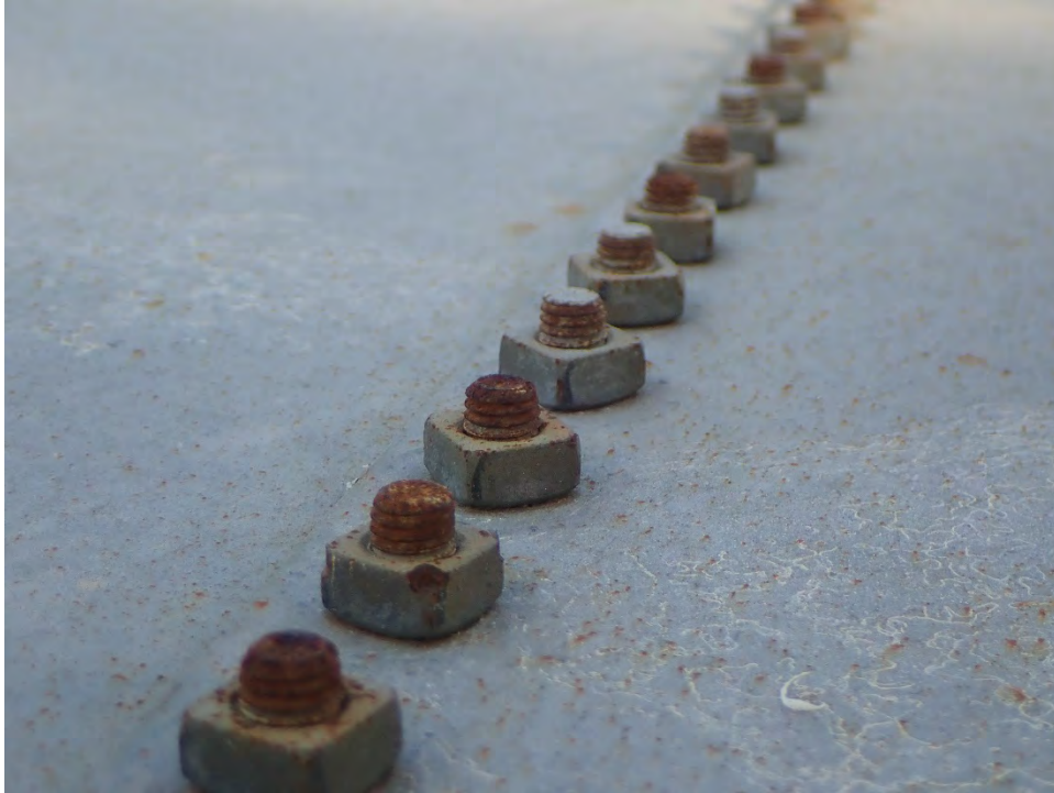
Photo 9: Roof with corrosion
