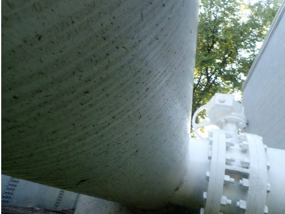
Photo 5: Piping with staining
