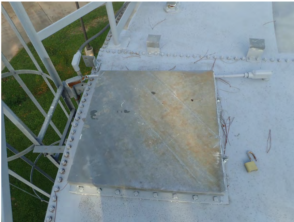
Photo 14: Roof hatch with corrosion
