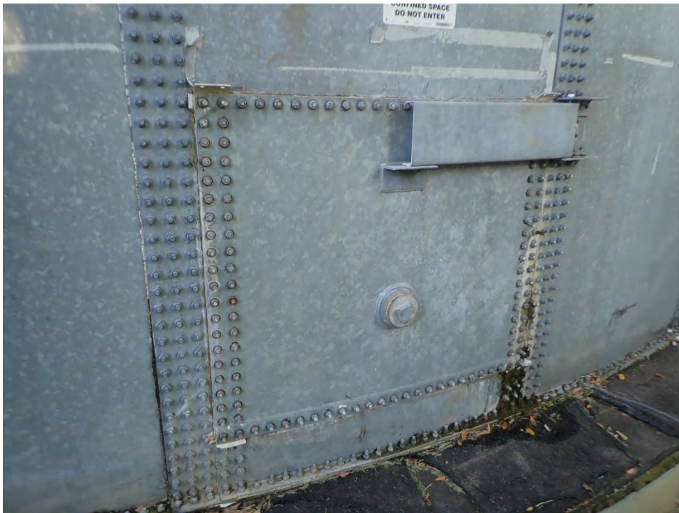
Photo 2: Side hatch with leak
