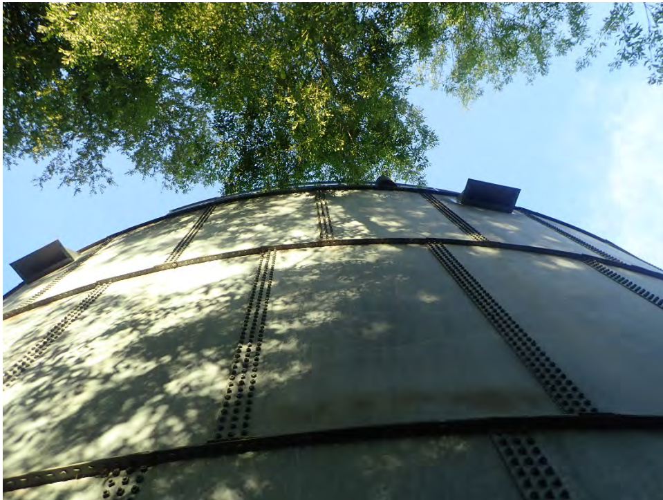
Photo 4: Sidewalls with tree encroachment
